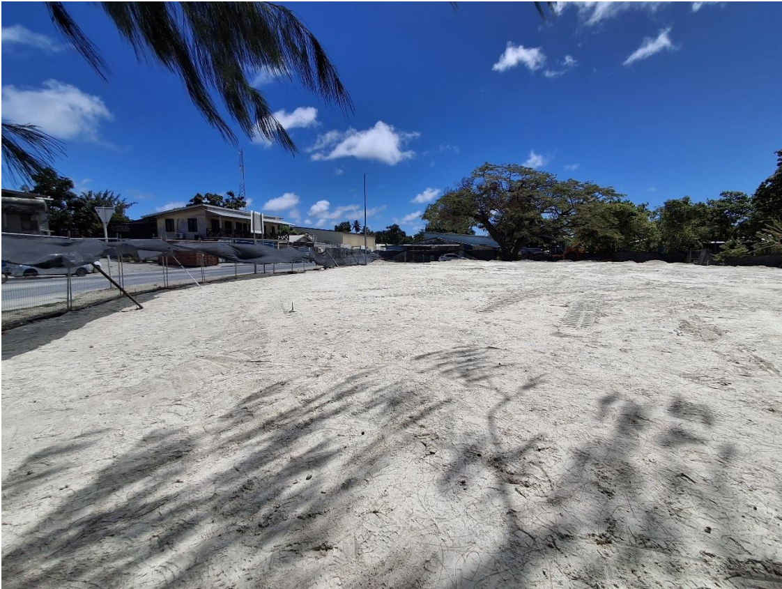
Figure 2: Completed early works condition on site (backfilling and compaction to formation level)
